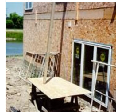
Scaffold in Dupage County
