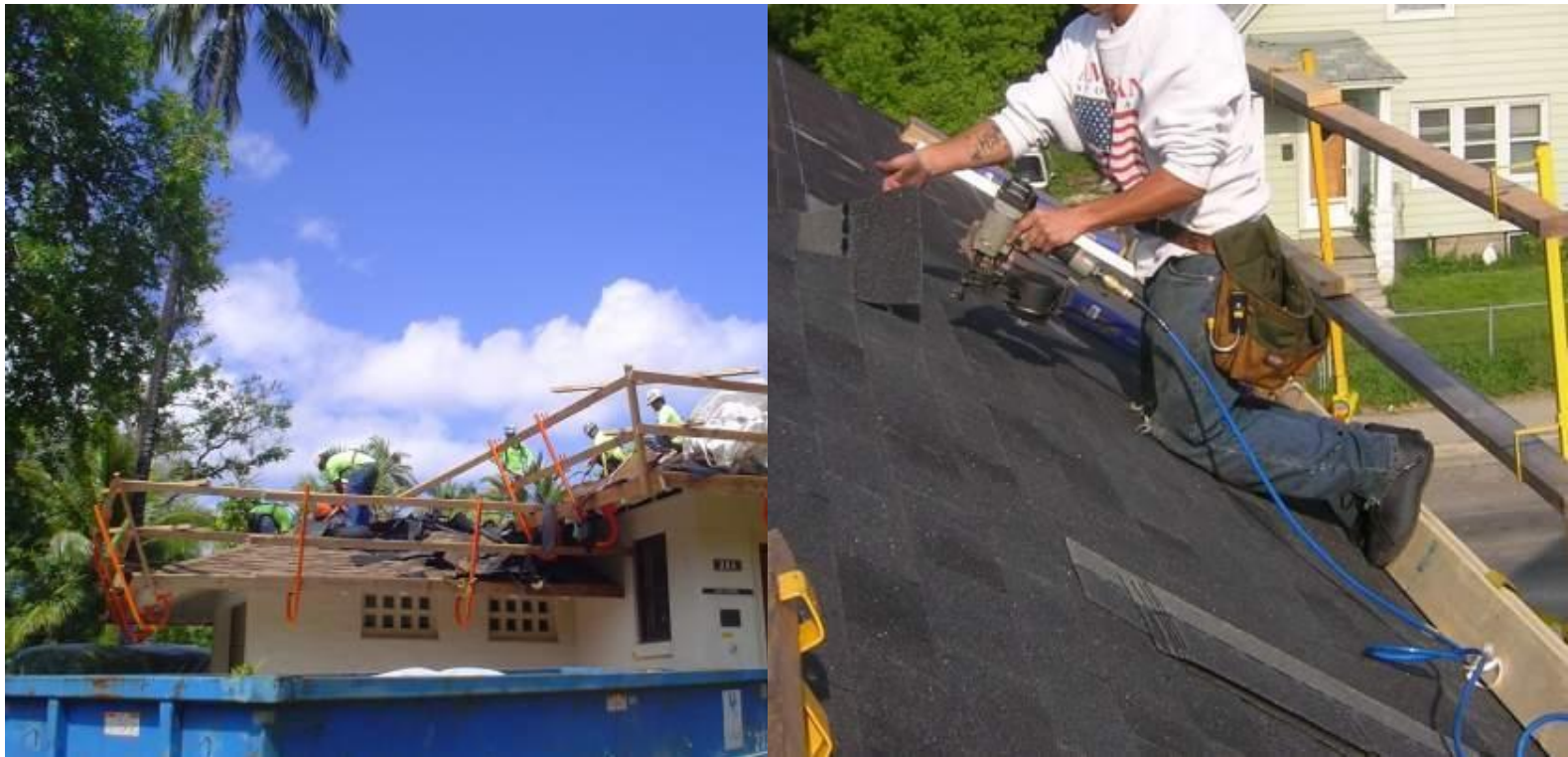
Guardrails in place during re-roofing activities.
